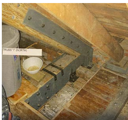
Roof truss repairs showing metal plates on both sides of the angle where the beam and truss are joined and are supported by the exterior wall.
