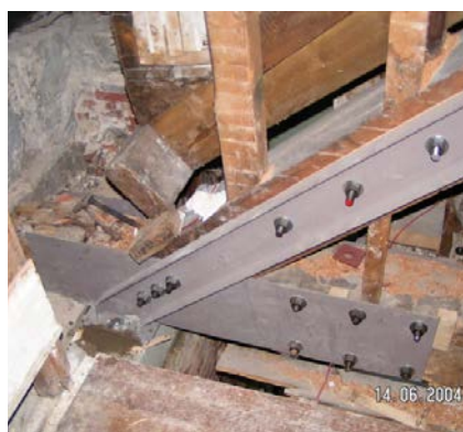
Roof truss repairs showing metal plates on both sides of the angle where the beam and truss are joined and are supported by the exterior wall.
